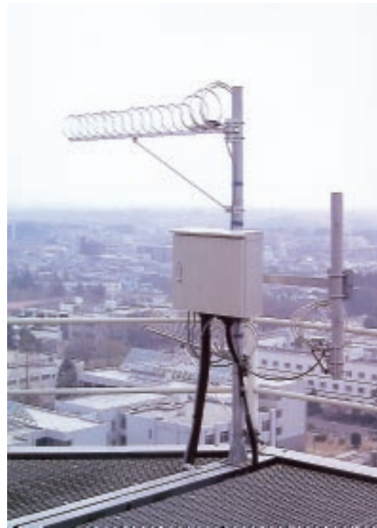
Digital terrestrial broadcasting antenna for experimental purposes
