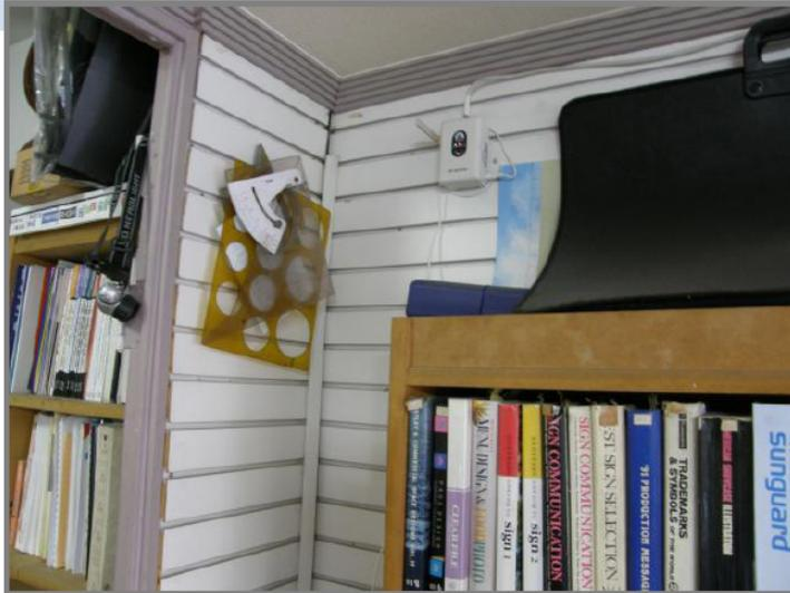
An RF SOHO Repeater is installed in an office where WiMAX signal can not reach inside.
