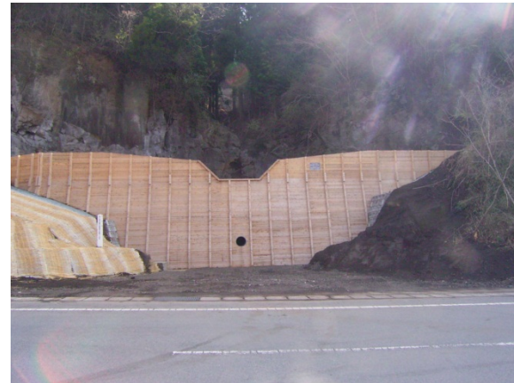
Wooden permanent form soil conservation facility constructed using local lumber (Ubuyama Village)
