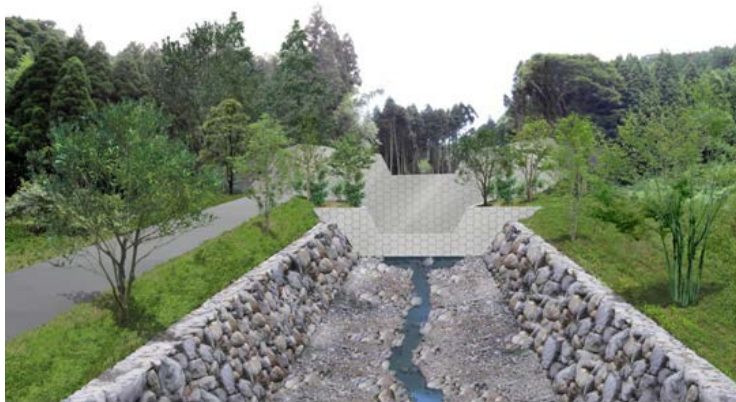
Erosion control facility using local stone (Aso City)
