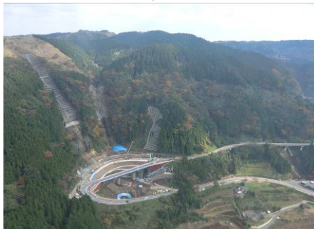
Disaster restoration works underway on the current road (Nov. 2013)
