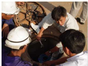
Water supply project at Phnom Penh
