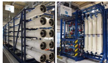
Seawater desalination system
