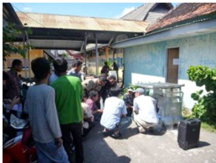
Installation of PVRO at a hospital on Sumbawa
