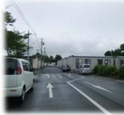
【Temporary housing outside town】
