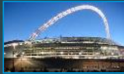
Wembley Stadium, London, UK
