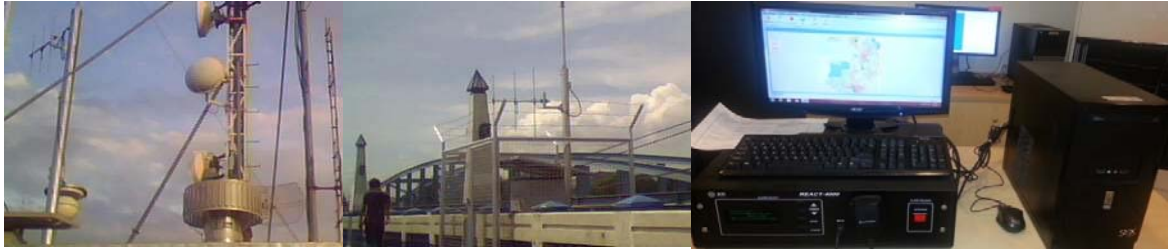
Wide Area Alarm Siren System
