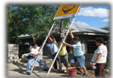
Installation of Flood Signages
