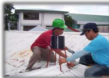
Setup of Digital Rain Gauge
