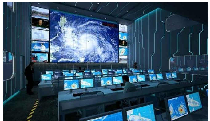
Image of Intelligent Operation Center (IOC)
