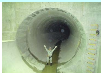
Large-diameter water pipe (3m~5m)
