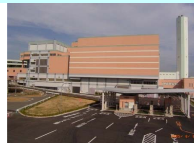
Tobu Incineration Plant
