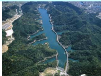
Construction a pump-up dam
