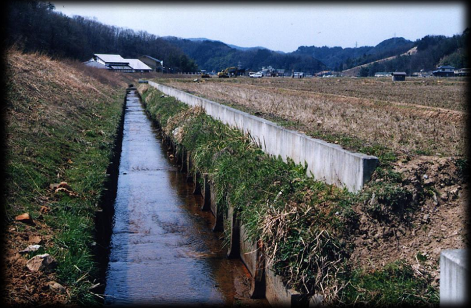
Soil was built up to create higher mounded rice paddies
