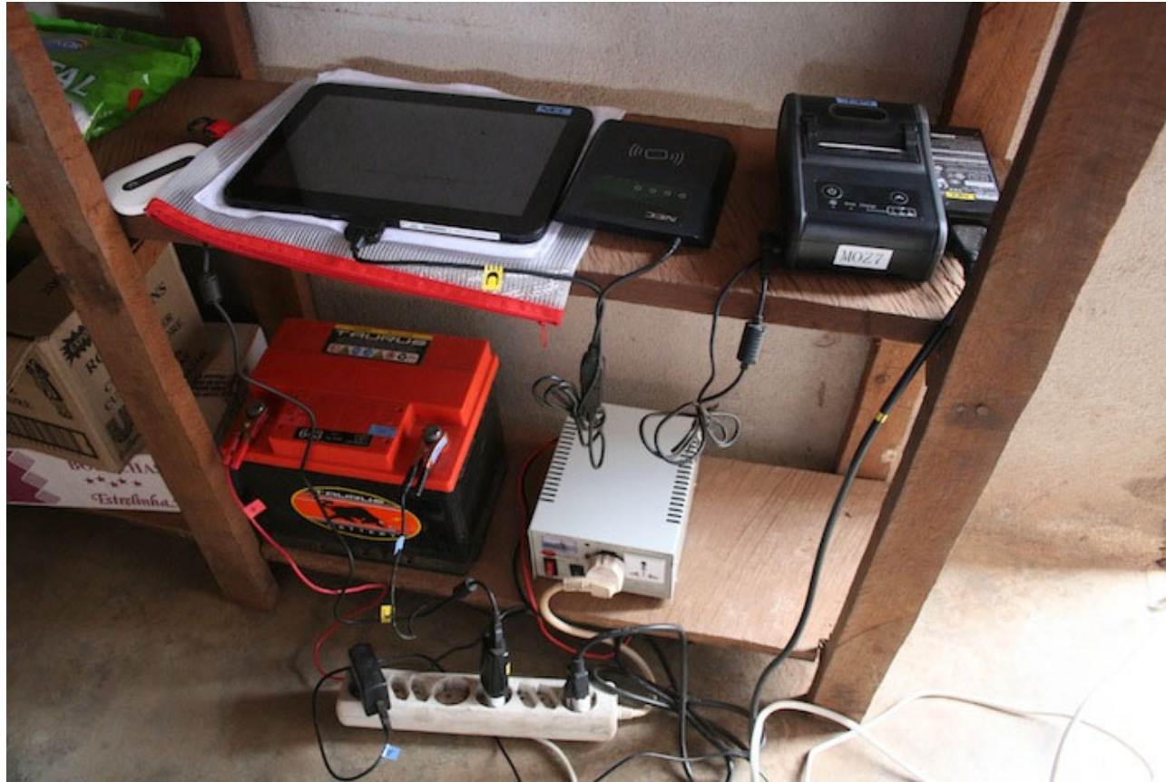
Equipment charged by solar panel
