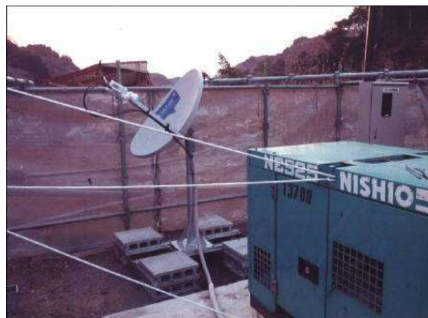
Satellite antenna installed -> service restored
