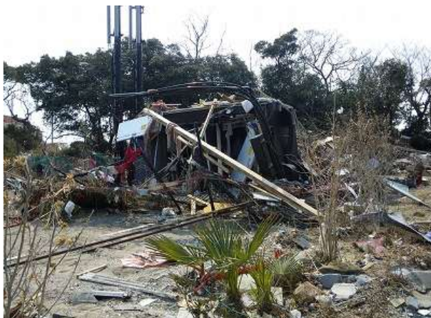
Damaged base station
