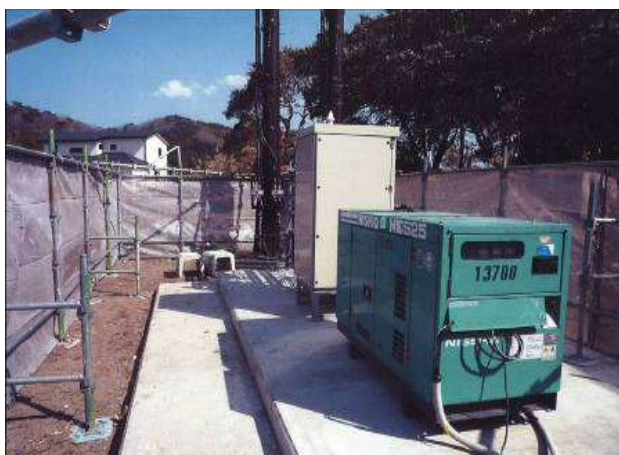
Installing radio and power equipment
