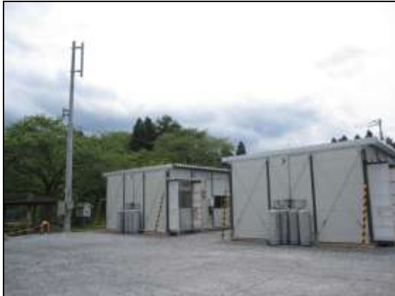
Improvements at temp housing area
