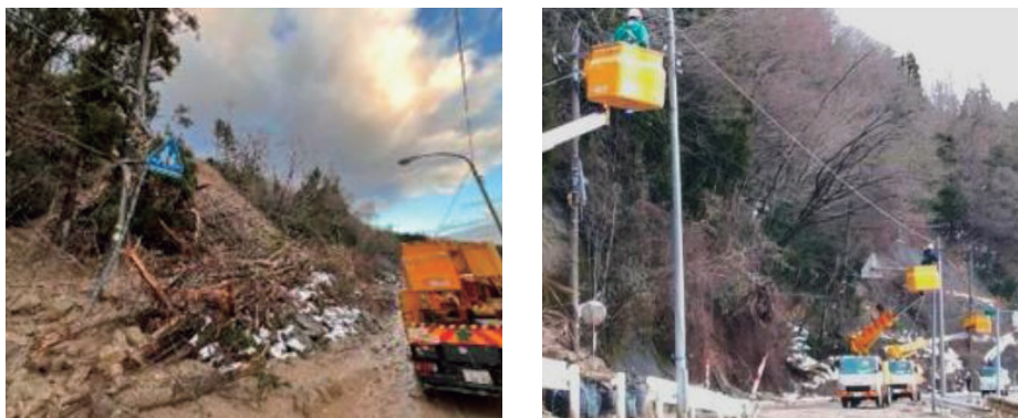
Figure 1-1-2-5 Damage to the communication infrastructure (mobile phones) (damage or replacement of optical fibers)
