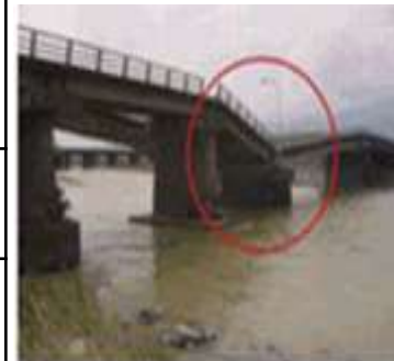
Subsidence of a pier
