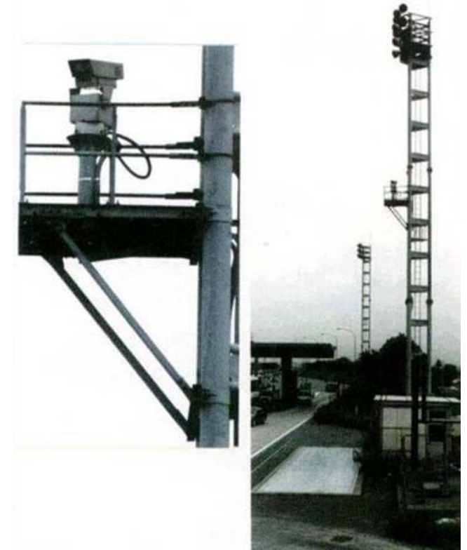
CCTV (Closed Circuit TV)
