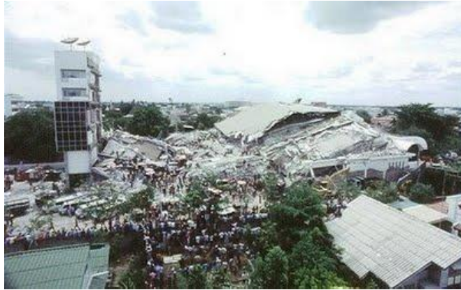
Royal Plaza Hotel collapse 1993
