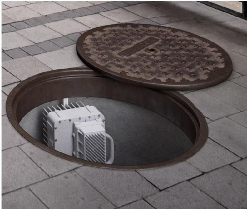
Underground vault sites
