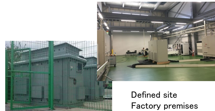
In situ Large equipment
