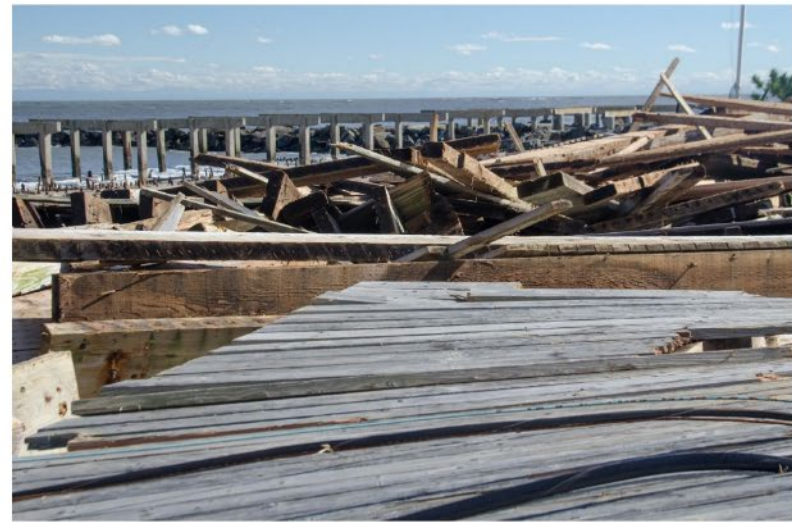
Damage to Atlantic City's Boardwalk Photo October 31, 2012 Photo by Liz Roll/FEMA より引用
