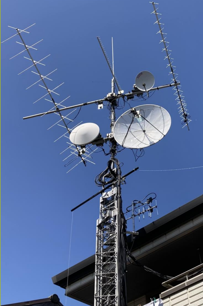
1.2m Dish 2.4GHz 25dBi LNA 30dB, Coax Loss -10dB
