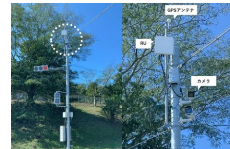
Installation of a device on a traffic light post
