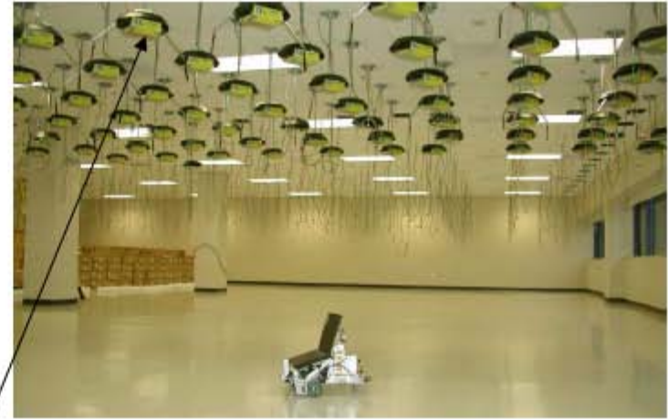
400-node radio grid system at Tech Center II (under construction 5/05)
